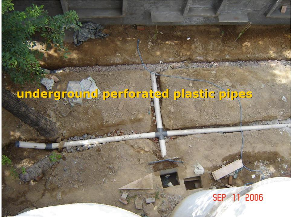
**underground perforated plastic pipes**
